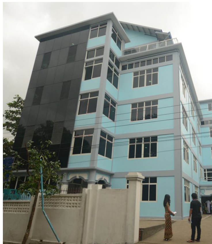
The first floor of the Anglican Training and Resource Center has classrooms, a study room, an office, and a community center. The second floor houses an upgraded library with multimedia and archive facilities. The third floor has classrooms and guestrooms. The fourth floor will have a graduation hall, community hall, and mini-theater.
